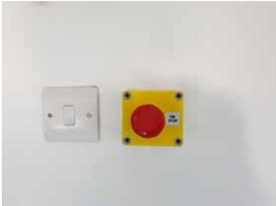
**IN CASE OF EMERGENCY**, push the red emergency shut off button, which will stop the flow of gas to the appliances.
